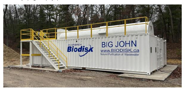
Packaged plants typically include primary treatment (settling), secondary treatment (biological), and sometimes tertiary treatment (filtration/disinfection), all within a compact footprint. RBC-based packaged plants, such as the <u>River Birch Biodisk</u>, offer a particularly robust and energy-efficient biological treatment process compared to other technologies.
